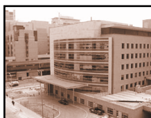
· The R. Fraser Elliot Building located at the north west corner of Elizabeth and Gerrard streets
